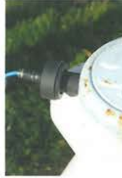
Listening at a hydrant with the magnet base
