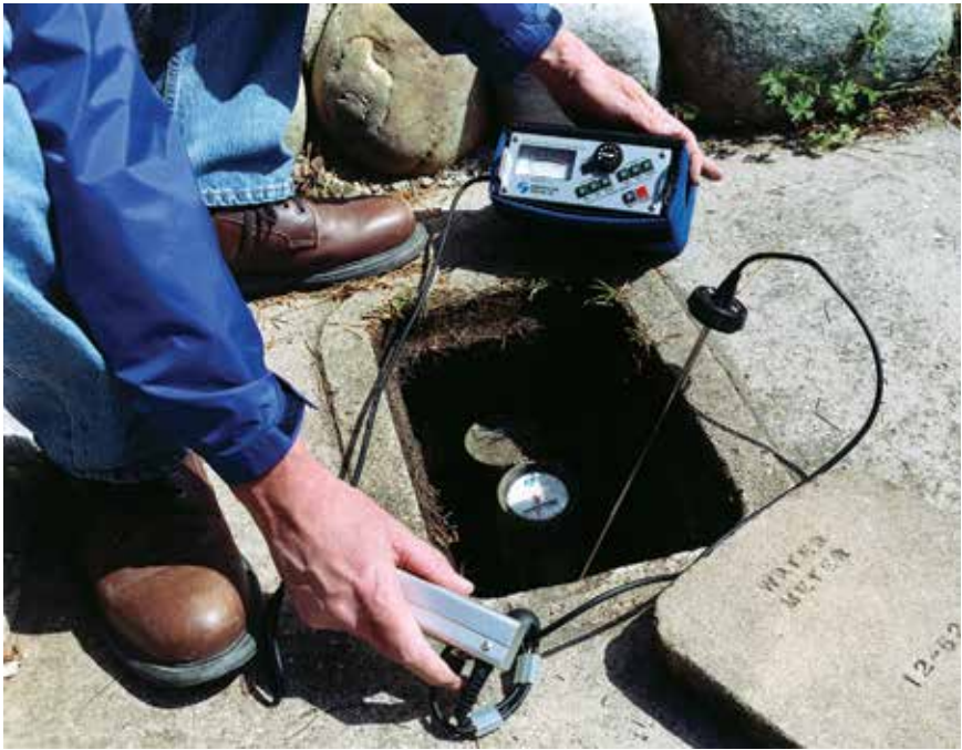
Figure 4-8 Leak Survey at a Meter
